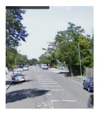
The major consideration of this feature is that, these markings can only be laid down the centre of roads which are 7 metres wide or more. They work on the principal of appearing to reduce the width of the running lanes. Speeding can therefore be inhibited to a degree, as overtaking will be discouraged.
