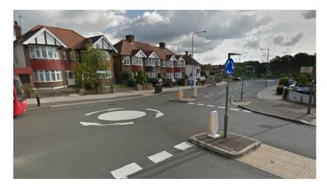
Mini roundabouts will have a calming effect but should only be installed in 20/30mph zones at three armed junctions, which have equal and/or substantial traffic flow on each approach. The mini roundabout itself must be greater than 1m in diameter but less than 4m and must not exceed 125mm in height.
